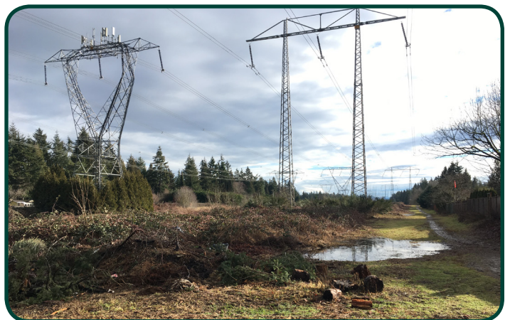
Site view from middle of site looking east.
