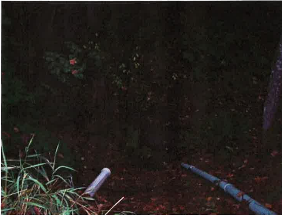
Photo 12: Pleasantdale Creek at Grade Crescent. Drainage pipes entering creek on downstream side of road
