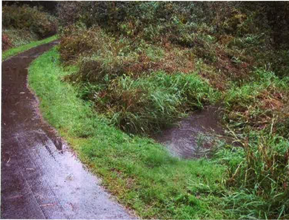
Photo 18: Langley Creek, pathway next to creek near Nicomekl River
