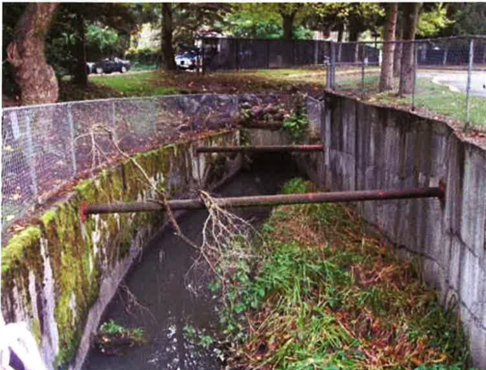
Photo 4: Baldi Creek, concrete lined section upstream of 55A Avenue
